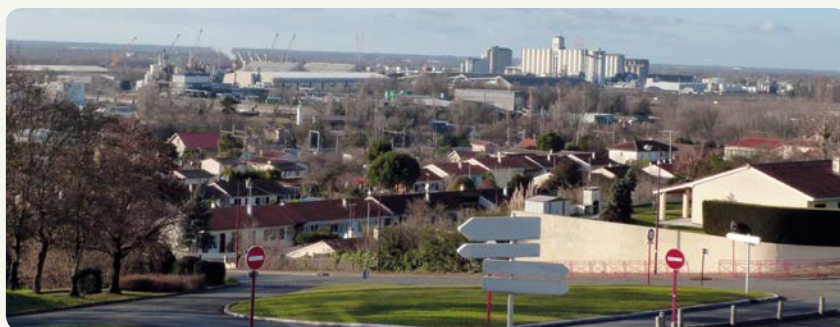
THE BASSENS INDUSTRIAL PORT AREA Photo: Bassens town hall
