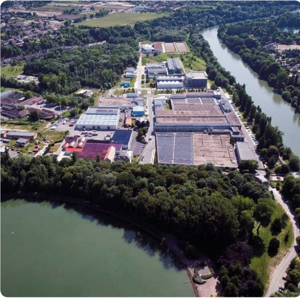
AERIAL VIEW OF SEDIF'S MÉRY-SUR-OISE PLANT Photo: SEDIF
