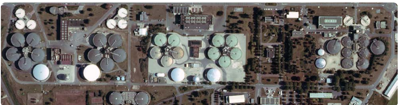
BIOGAS PRODUCTION : DIGESTERS CLUSTERS AND GASOMETERS OF THE SEINE AVAL WASTEWATER TREATMENT PLANT
