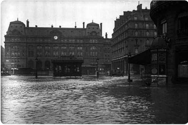
FLOODS IN PARIS ON 28 JANUARY 1910. COUR DE ROME AND PLACE GABRIEL PÉRI, SAINT-LAZARE STATION
