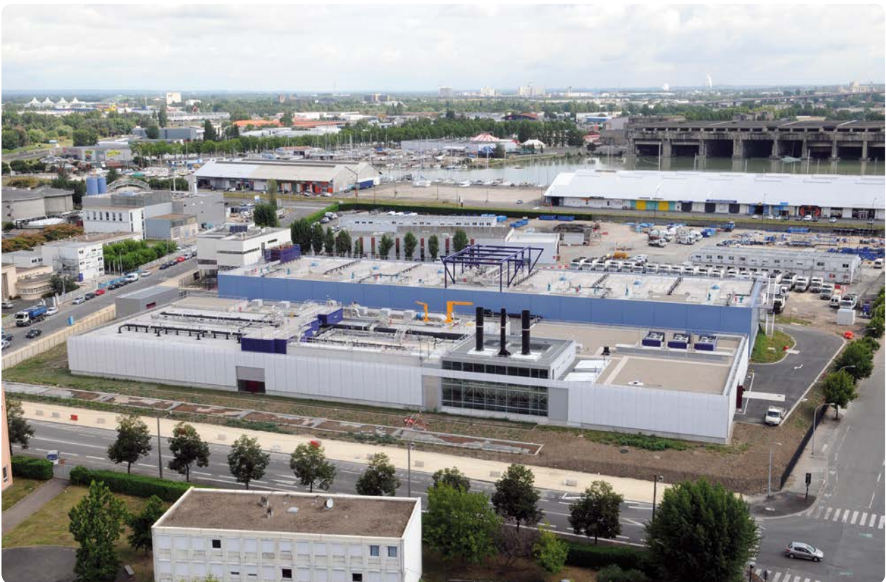
THE LOUIS FARGUE TREATMENT PLANT (JULY 2012)
