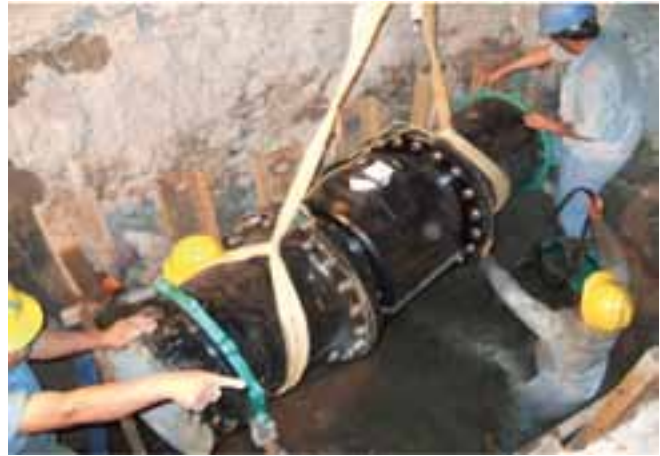
Installation of electromagnetic flowmeters
