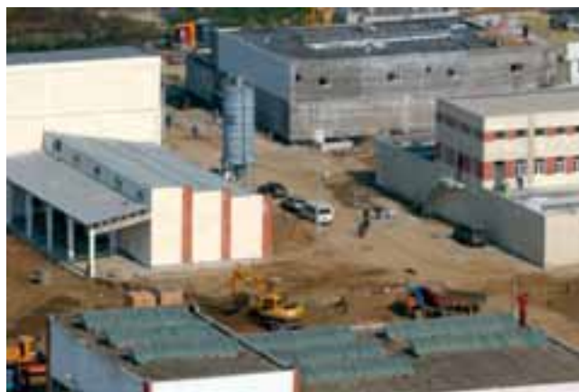
Crivina WTP during construction works (in operation from June 2006)
