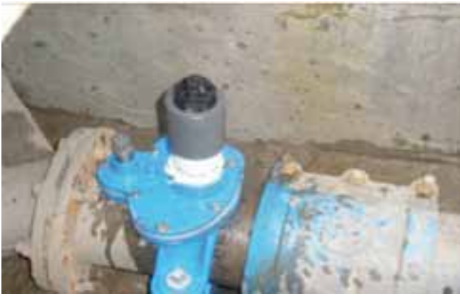
Kapta probes allow for continuous quality parameter measurements
