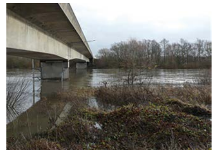
Hydrometric station of Hagondange on the Moselle River: water height measurement with two radar sensors under a road bridge
