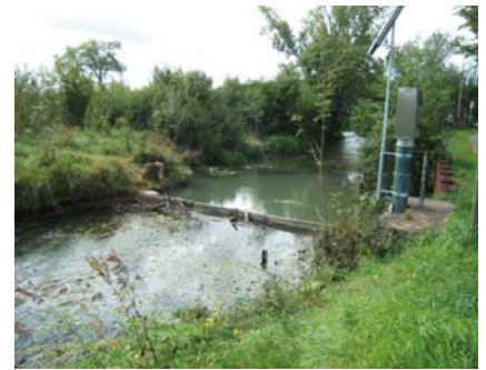
Water level station with solar panel upstream of a weir
