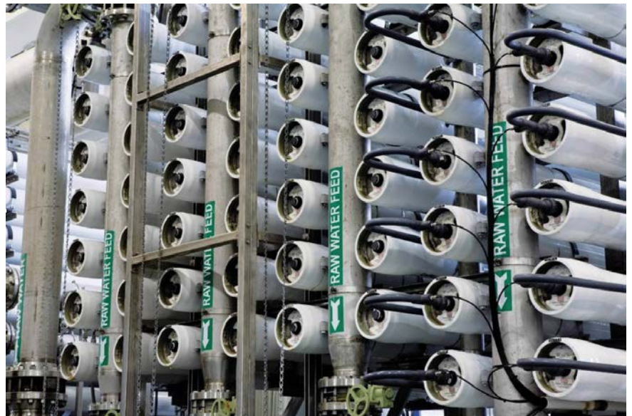
55% of Malta's drinking water comes from sea water desalinated by reverse osmosis
